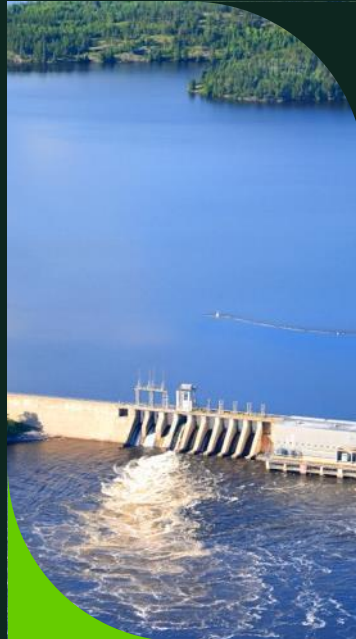
Investing in new and existing hydro
